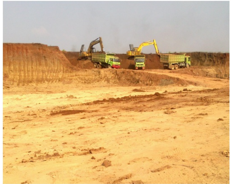
Cut and Fill Work in Phase 3
